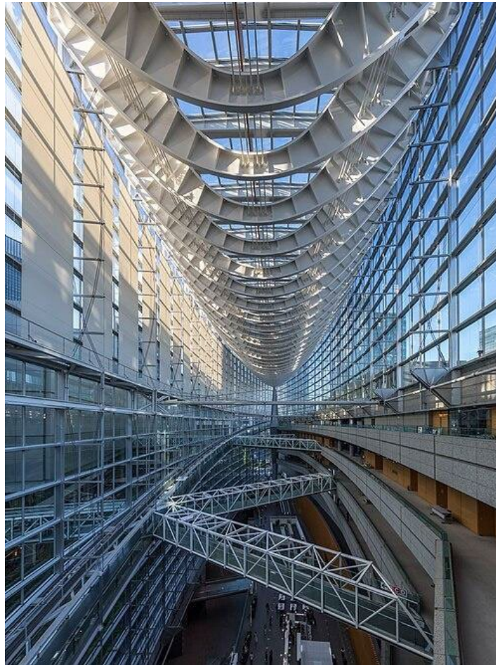
Figure 10. Tokyo International Forum Glass Hall: steel trusses, glass enclosure and public bridges. Photograph by Basile Morin, Wikimedia Commons, CC BY-SA 4.0.
