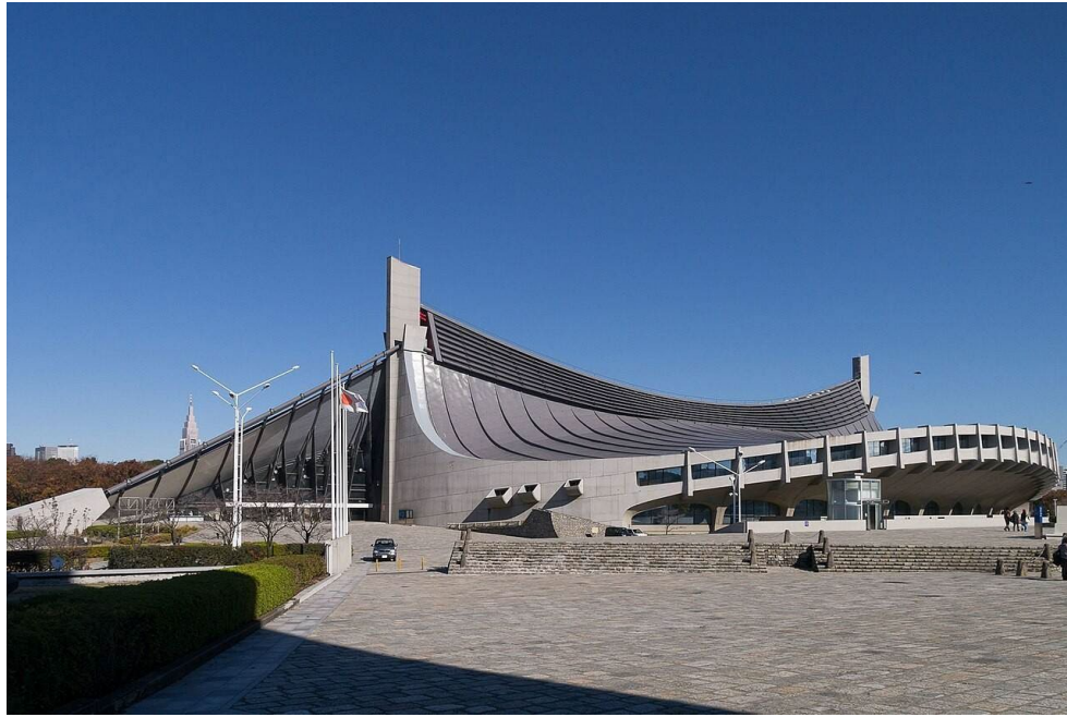
Figure 5. Yoyogi National Gymnasium, Tokyo: Tange's suspension roof makes structure spatially expressive. Photograph by Rs1421, Wikimedia Commons, CC BY-SA 3.0.
